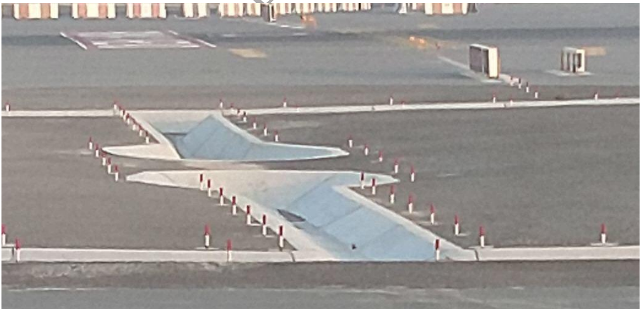
Drains at Dubai Airport with Marker poles
